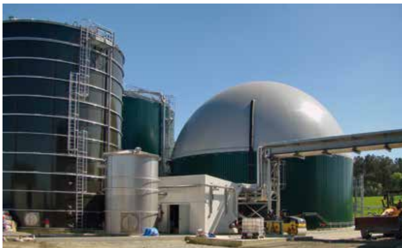
Territorial and collective biogas unit, Le Mené (France)
