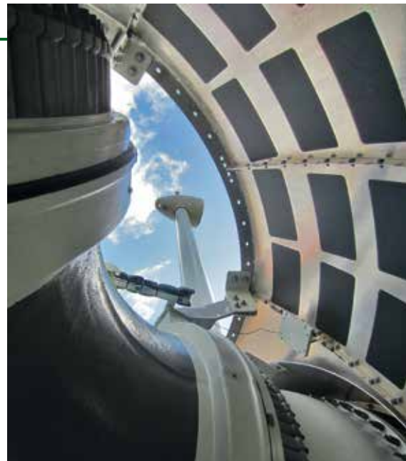
Wind turbine implementation, PSDT project (Scotland)
