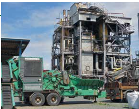
Biomass gasification plant, Güssing (Austria)
