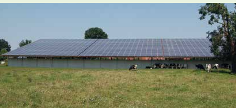
Solar farm, Osnabrück (Germany)
