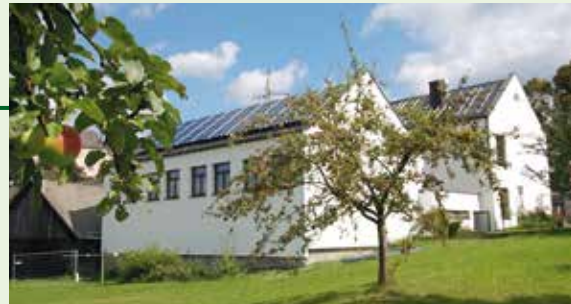
Thermal insulation, School Albrechtsberg (Austria)
