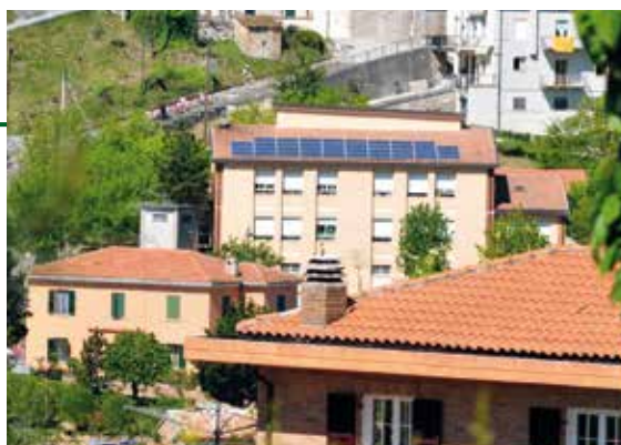
Photovoltaic plant on roof of school (Italy)
